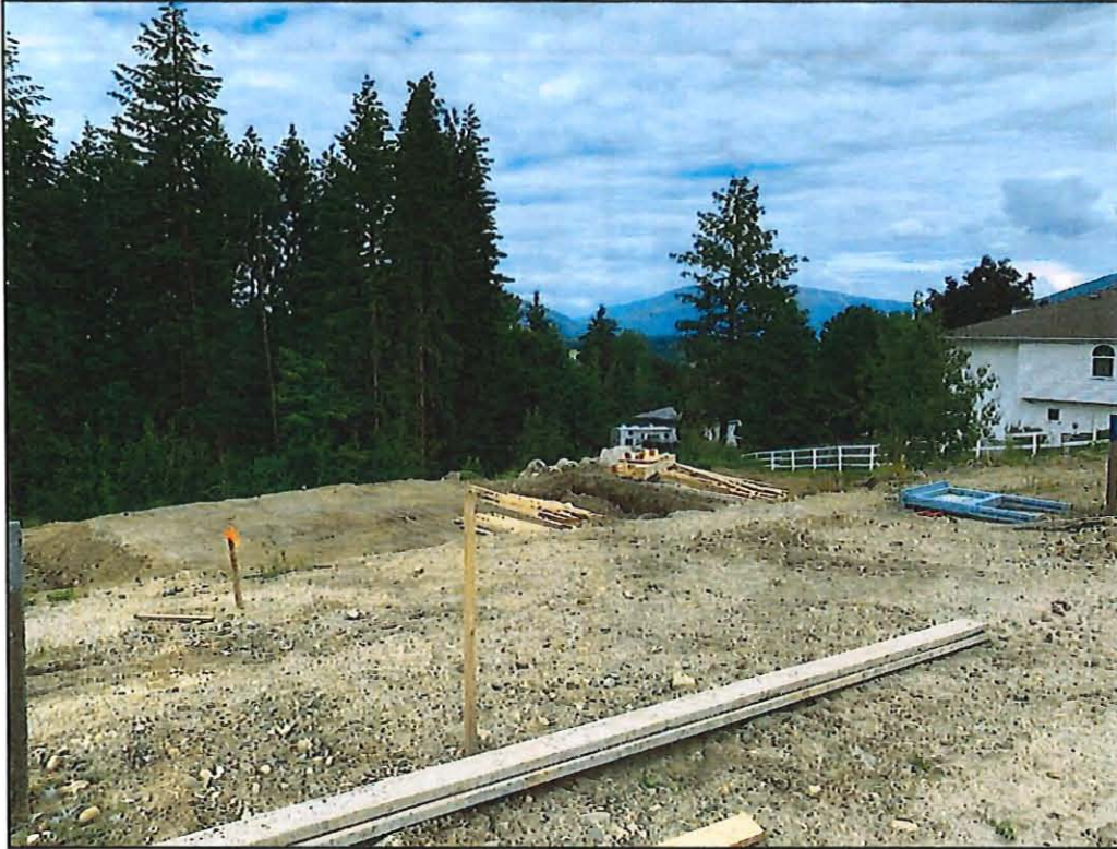
View of subject property looking southeast
