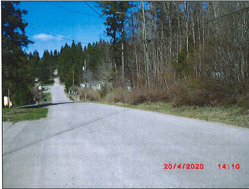
11 Street SE Looking North
