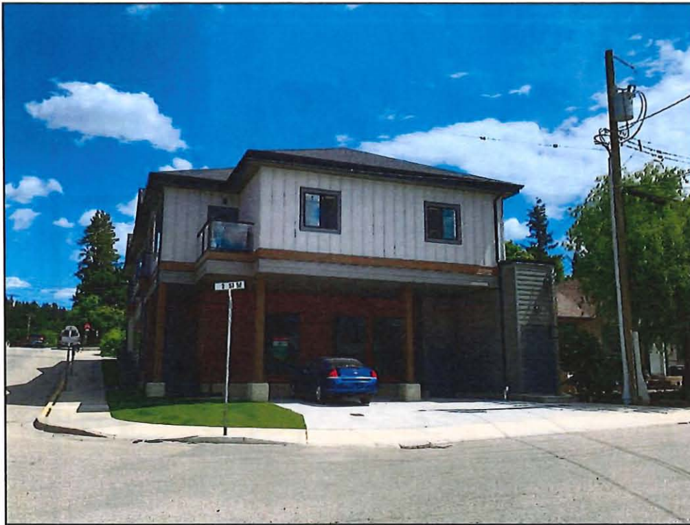
View of subject property looking east (from 2 nd Street SE)
