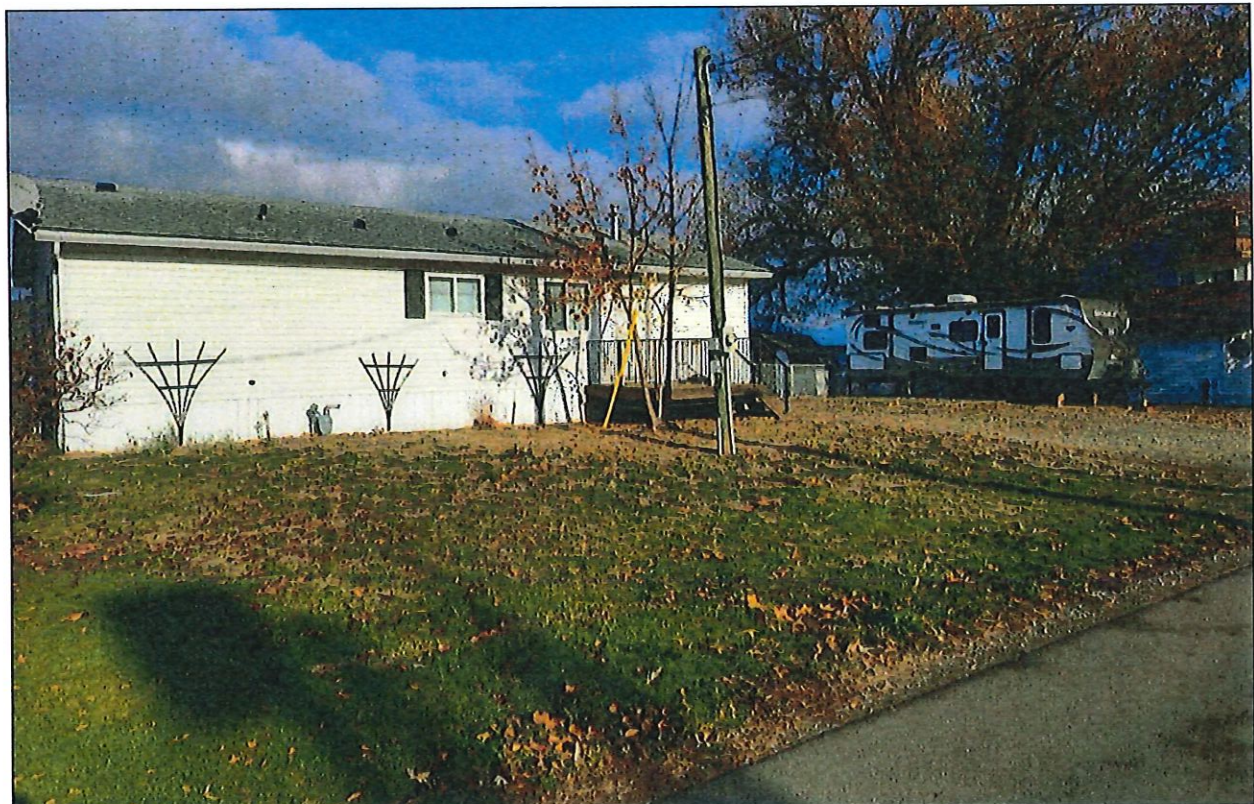
View of subject parcel looking northeast from 75 Ave NE.
