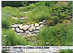
IMG 01: EARTHEN & CORBIE CHECK DAM
