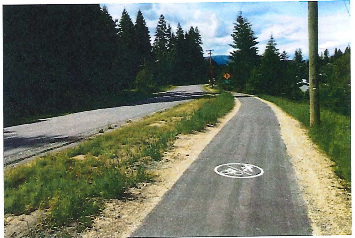
Salmon River Road Parallel Path (Silver Creek) – CSRD Area D
