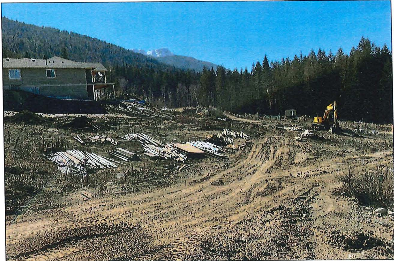
View of subject parcel south from 15 Avenue SE.
