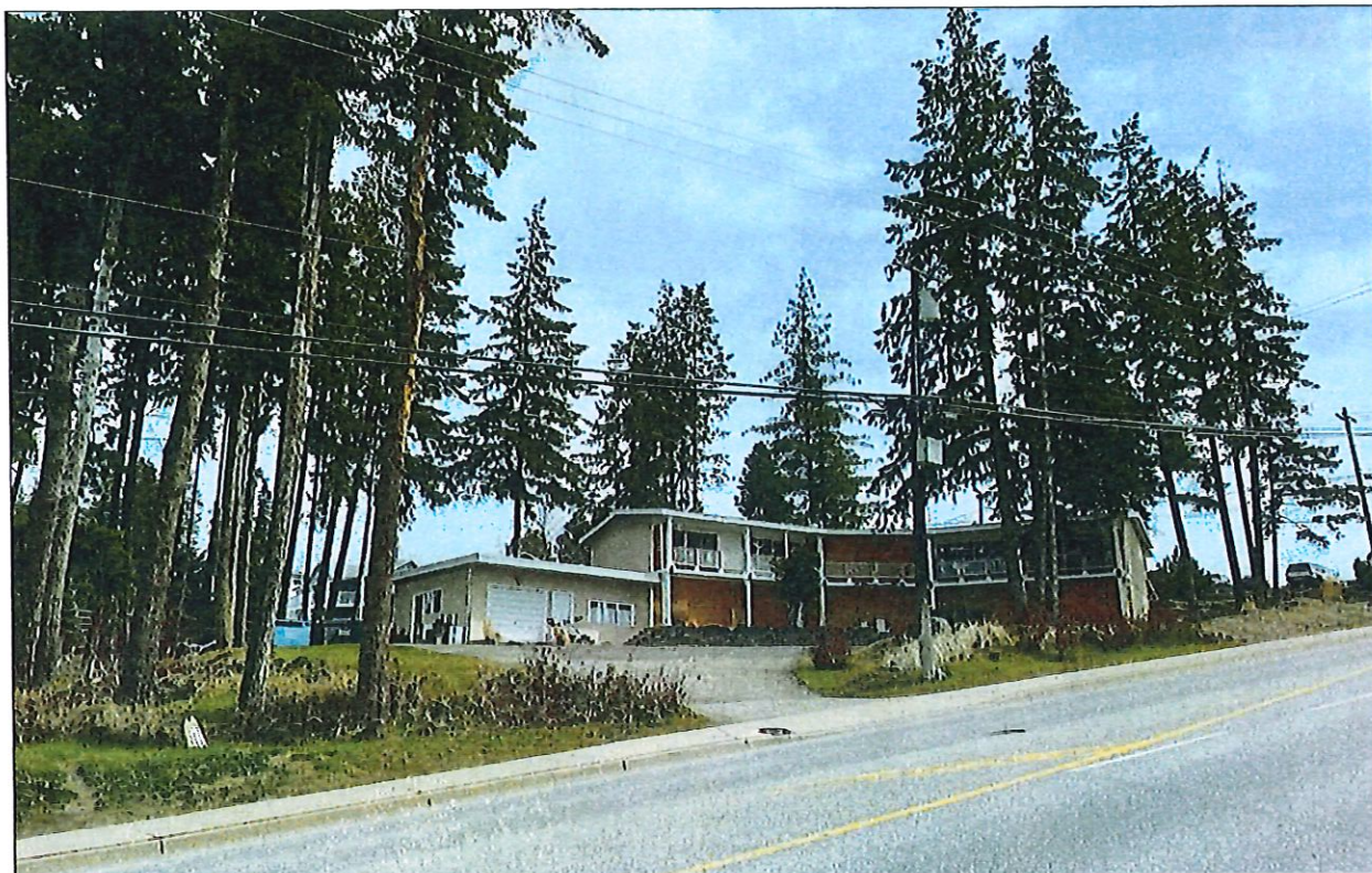
View southeast from 30 Street NE.
