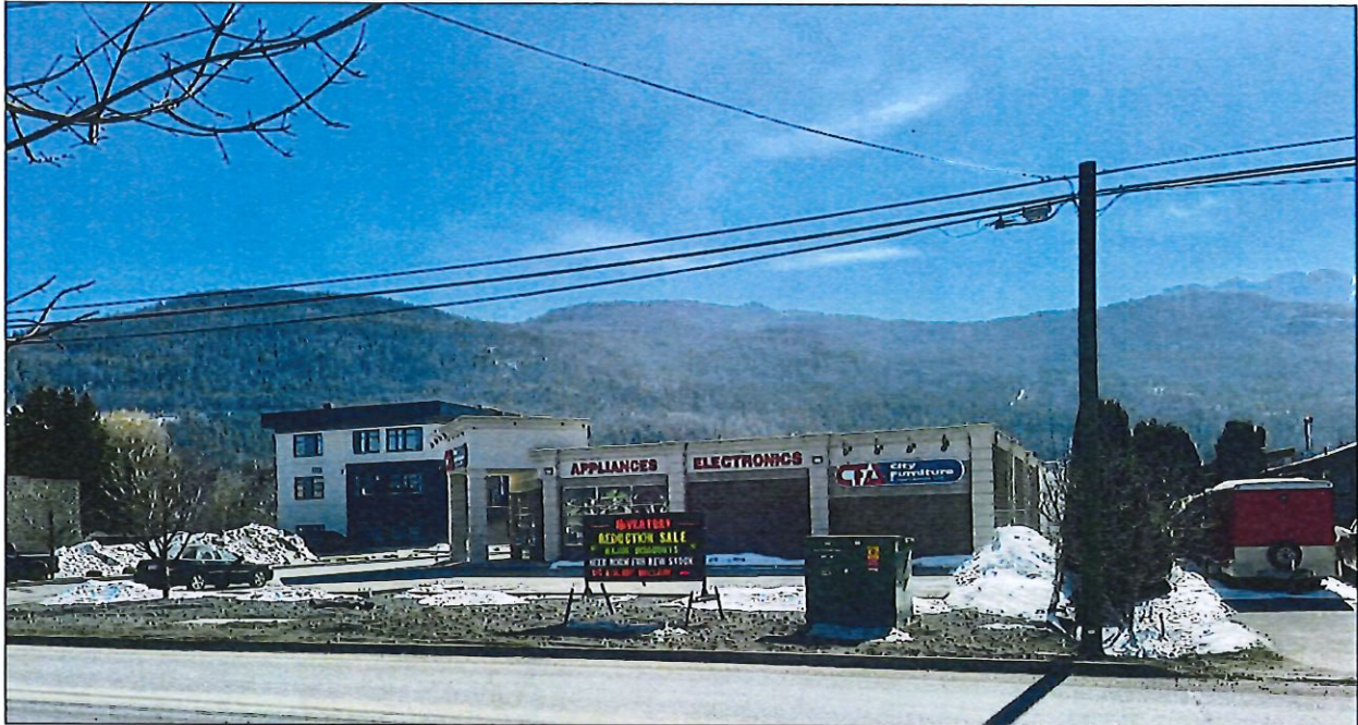
View of subject property southeast from 10 Avenue SW.
