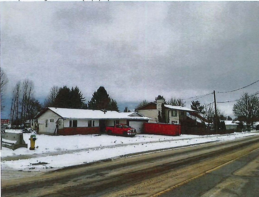
Photo 2: photo looking northwest at subject property and 10 Street SW
