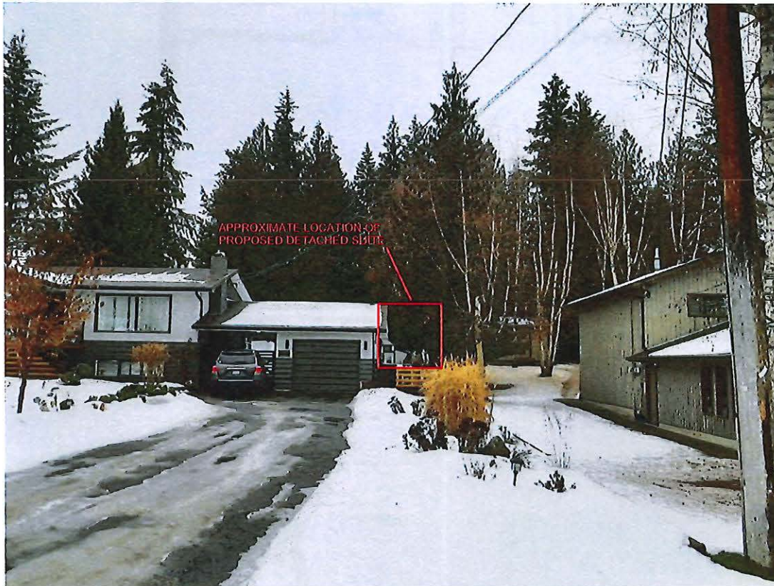
Photo 2: photo looking north at existing single family dwelling and attached carport/garage
