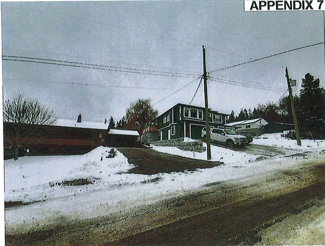
Photo 1: photo looking northeast at 25 Avenue NE, subject property and neighbouring property
