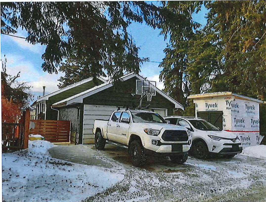
Photo 4: photo looking northwest at subject property
