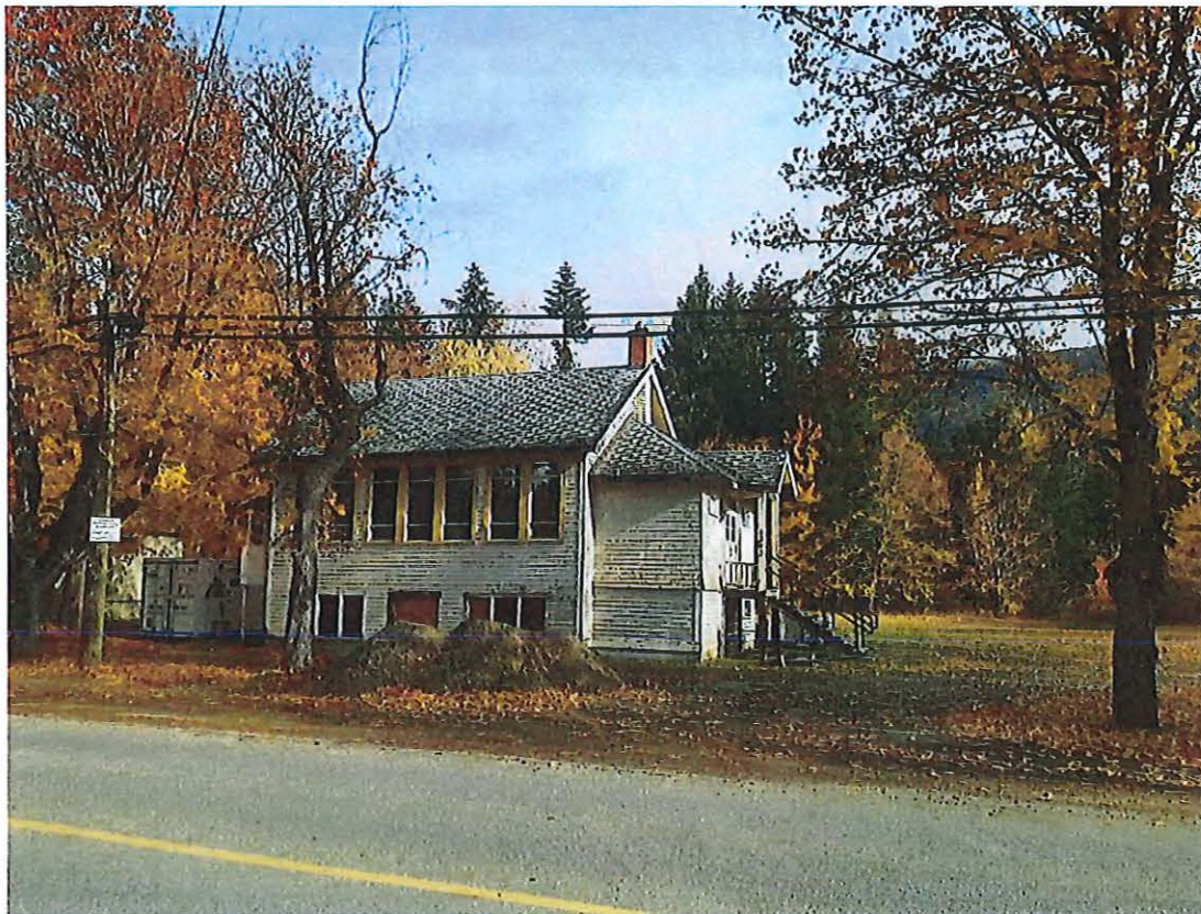
Photo 2: photo looking east at existing building/structure and 50 Street NE
