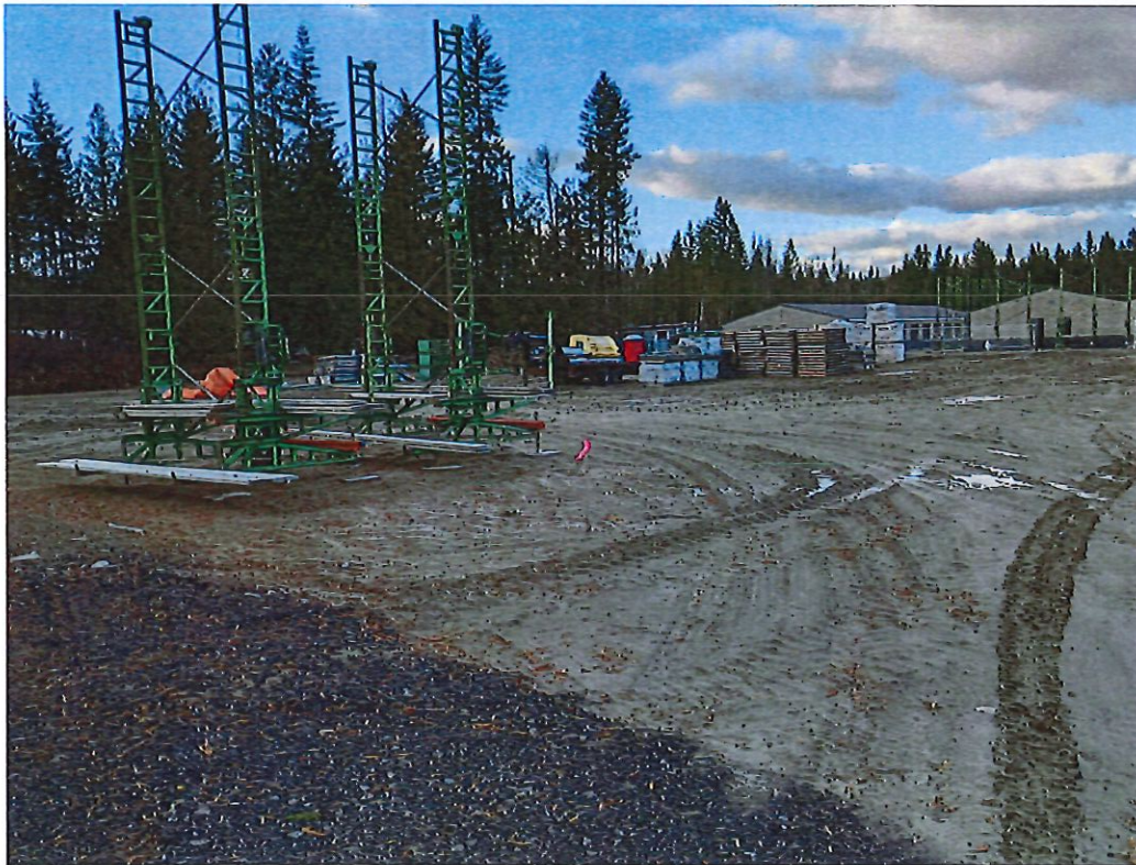
View northwest near southeast corner of subject parcel
