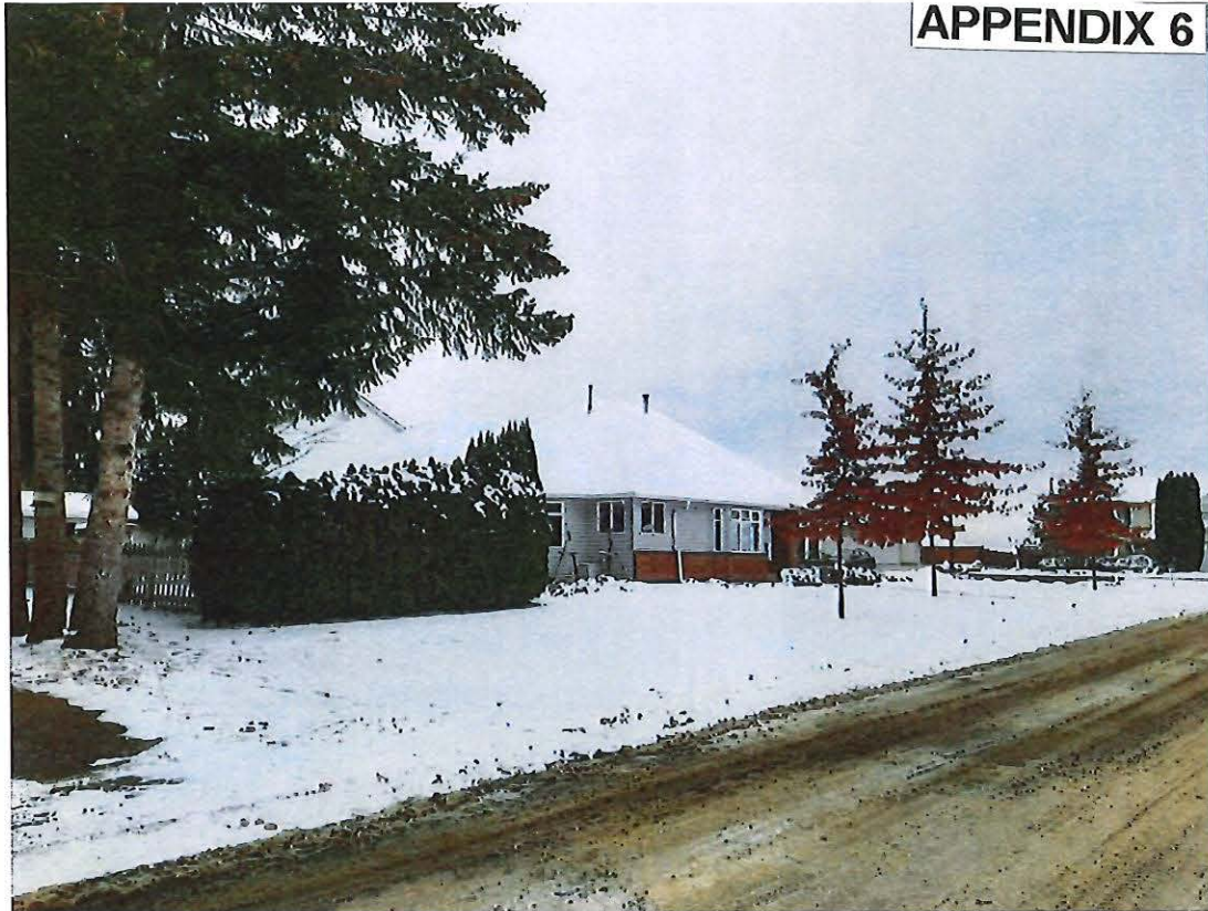
Photo 1: photo looking northwest at subject property and 25 Street SE
