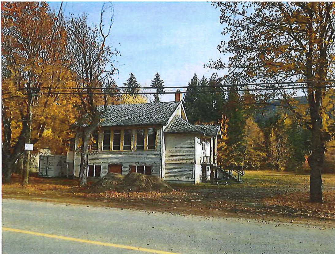
Photo 2: photo looking east at existing building/structure and 50 Street NE
