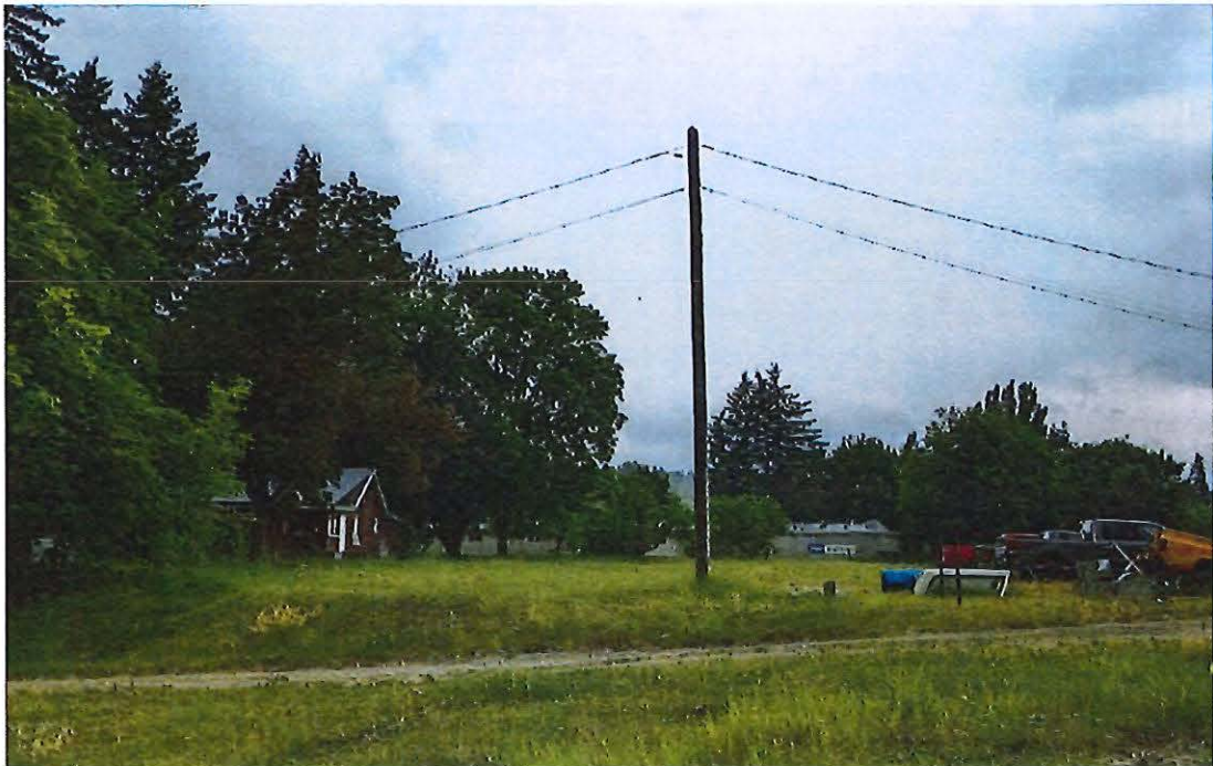
Near build site looking west.
