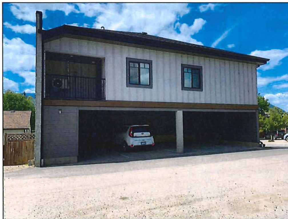
View of subject property looking west (from laneway)
