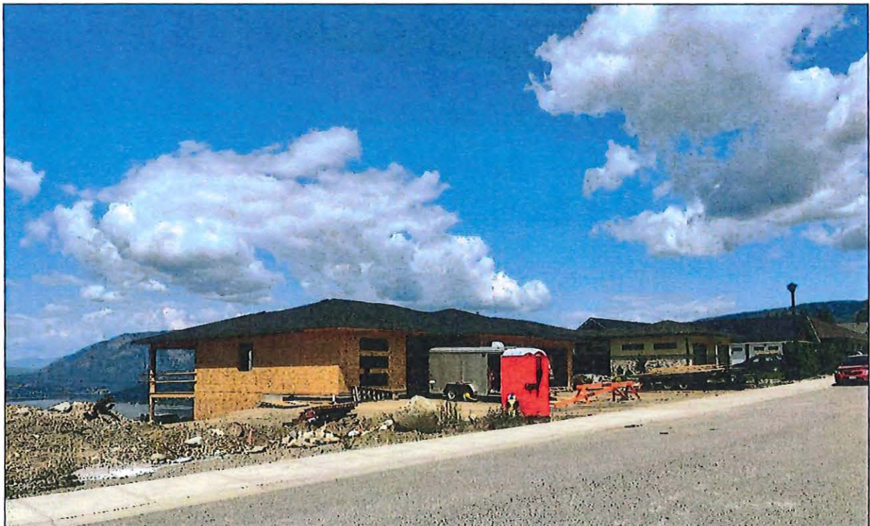
View northeast of subject parcel from 19 Avenue SE
