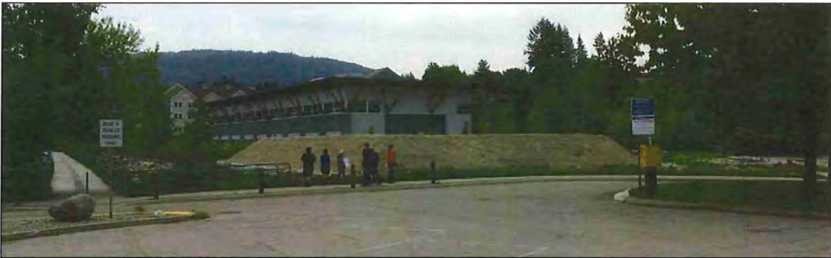
View east of subject property.
