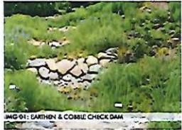
IMG 01: EARTHEN & COBBLE CHECK DAM
