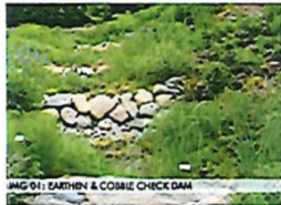
IMG 01: EARTHEN & COBBLE CHECK DAM
