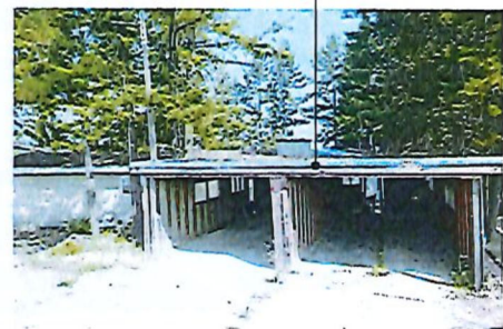
EXISTING CARPORT - TO BE REFINISHED
