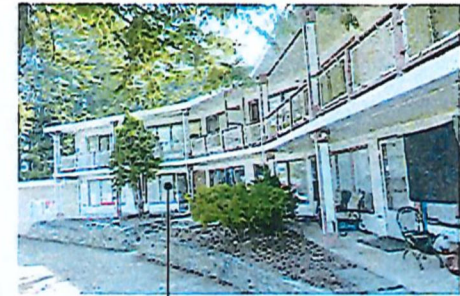
EXISTING RESIDENTIAL BUILDING - TO BE REFRESHED AND MODIFIED AS PER FLOOR PLANS & ELEVATIONS
