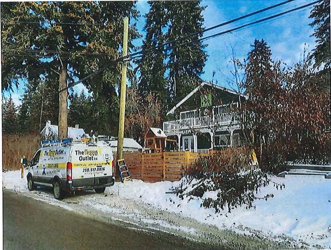
Photo 2: photo looking northeast at subject property
