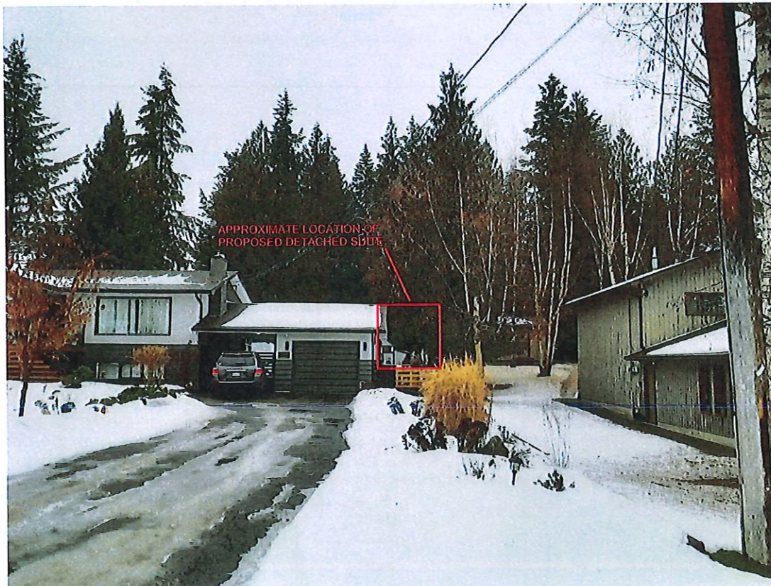
Photo 2: photo looking north at existing single family dwelling and attached carport/garage
