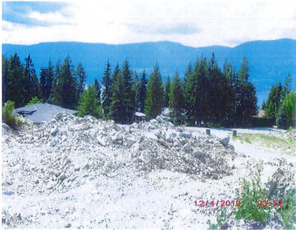
View looking west towards 20 th Street NE
