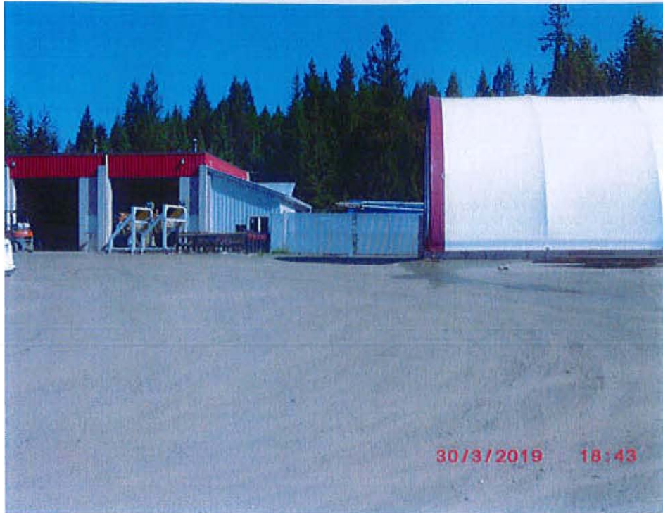
T-1 Enterprises, new fabric structure shown on the right
