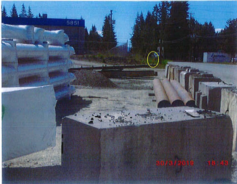
Facing southeast, showing the hydrant on Auto Road SE, southeast of the subject properties
