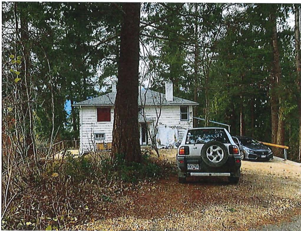
View of subject property looking northwest.
