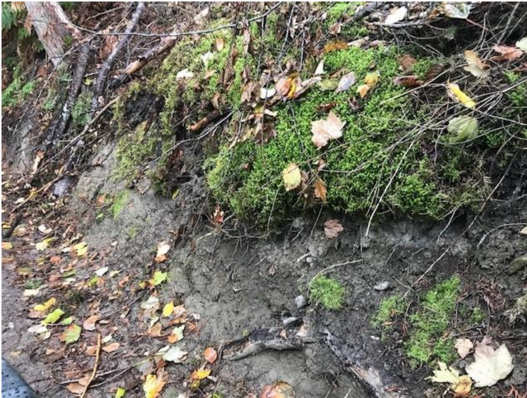
Photograph 2: Cut showing the Parent Clay Material
