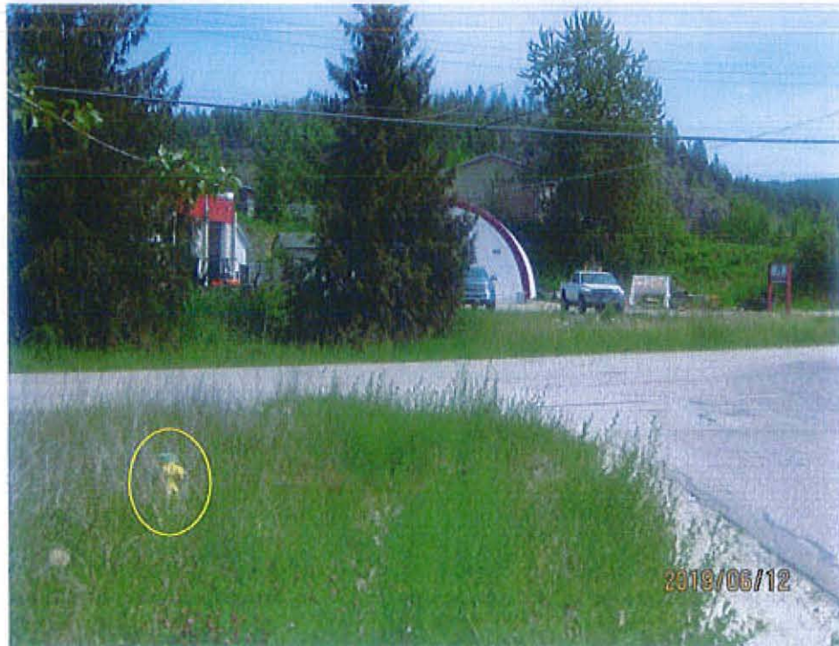
Facing east towards T-1 Enterprises, showing the fire hydrant at the intersection of 46 Avenue & Auto Road SE
