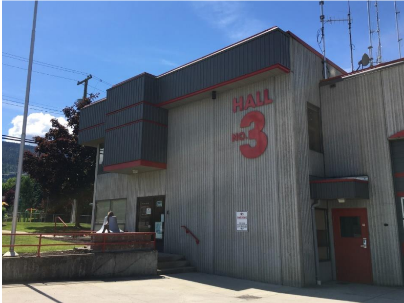
Figure 24: Fire Hall No.3 Building
