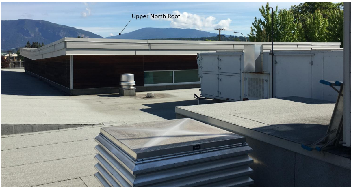
Figure 3: City Hall Upper North Roof
