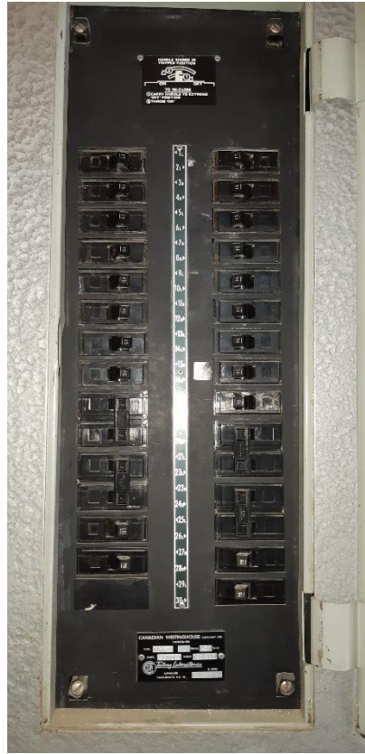
Figure 49: Art Centre Main and Sub Panels – No Spare Breaker Positions
