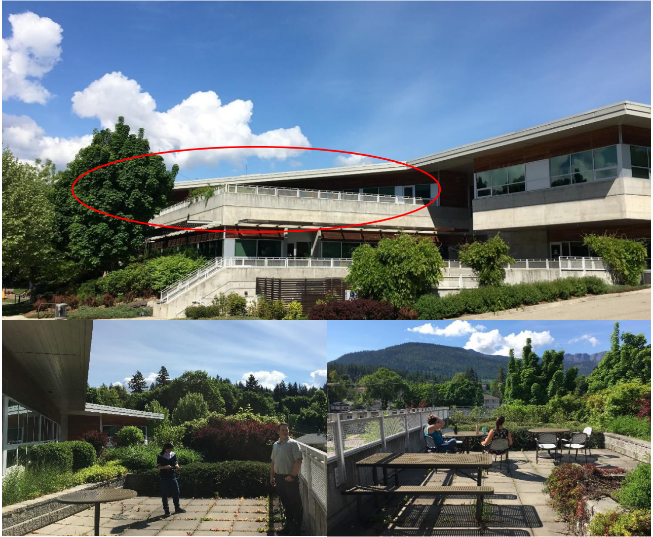
Figure 16: Level 2 South Patio Areas
