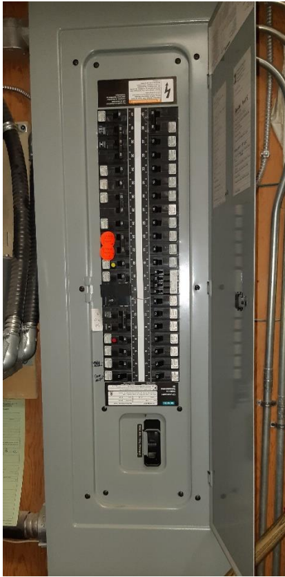
Figure 49: Art Centre Main and Sub Panels – No Spare Breaker Positions
