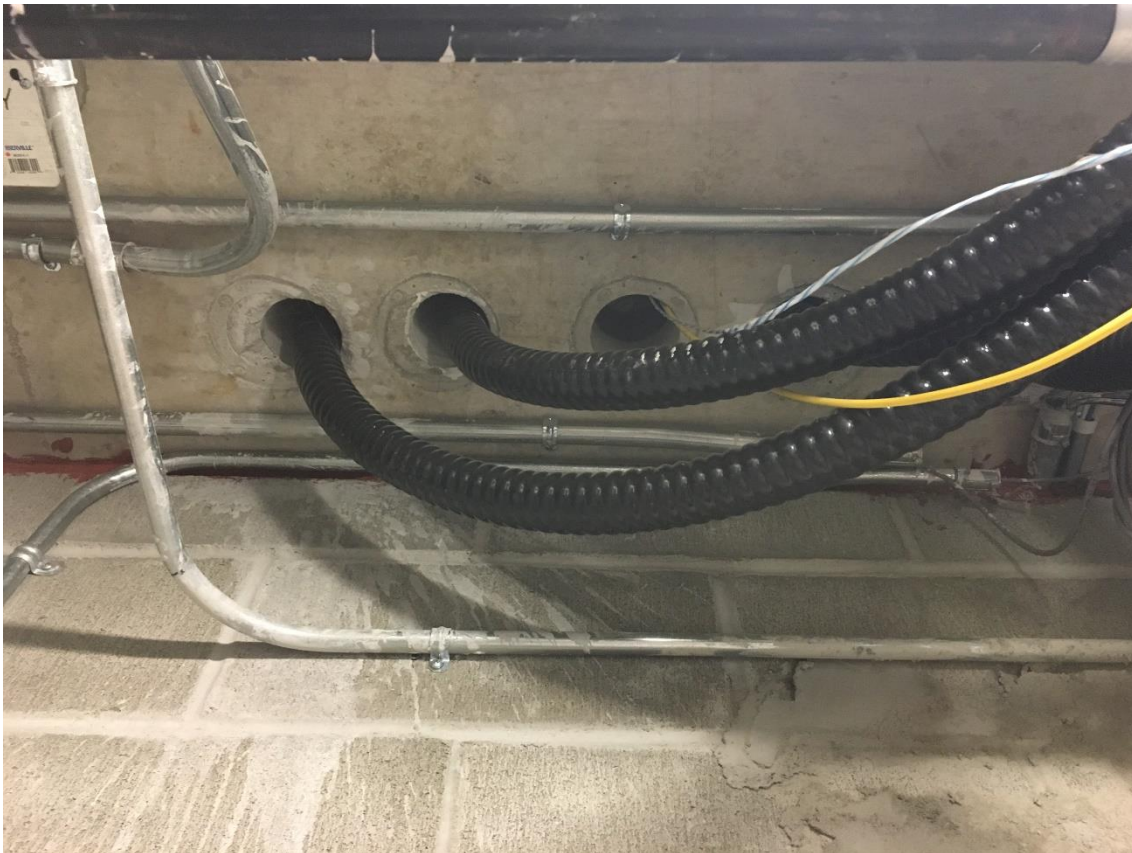
Figure 20: Electrical Cable Ceiling Slab Cores – Main Electrical Room 004
