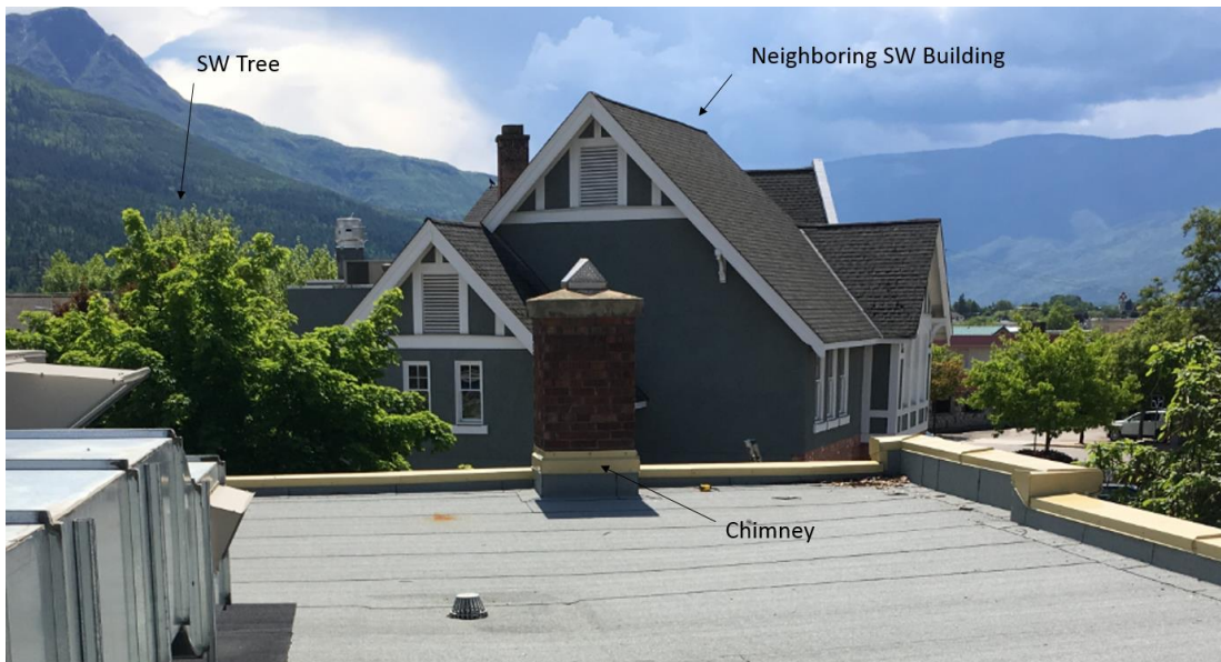
Figure 45: Art Centre South West Roof Shading Obstructions
