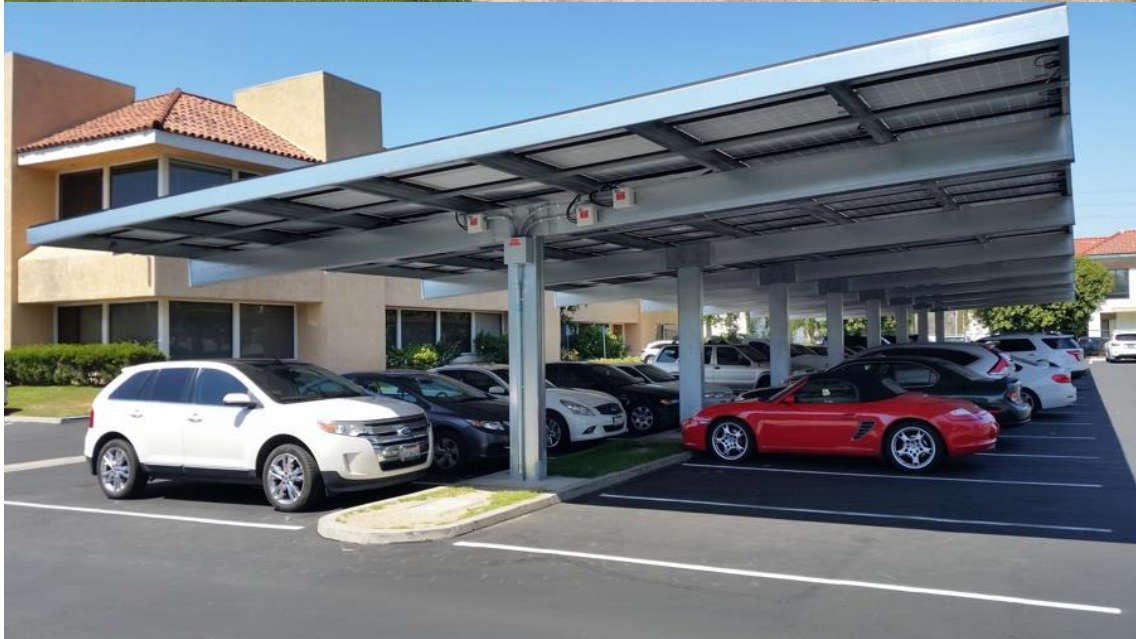
Figure 18: City Hall South Parking Area and a Solar Parking Shelter Example
