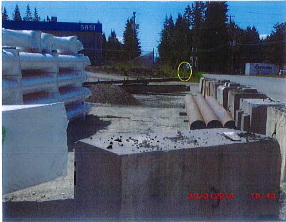
Facing southeast, showing the hydrant on Auto Road SE, southeast of the subject properties
