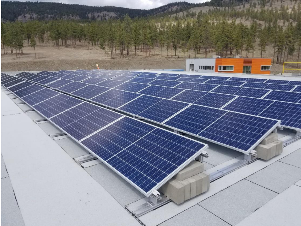
24.5 kWp Array using Ballasted Racking – Nicola Valley Institute of Technology, Merritt BC
