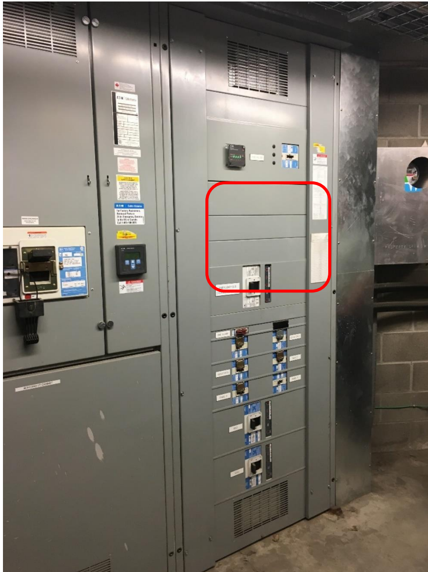
Figure 21: MDC - Room 004 – Spare Breaker Positions
